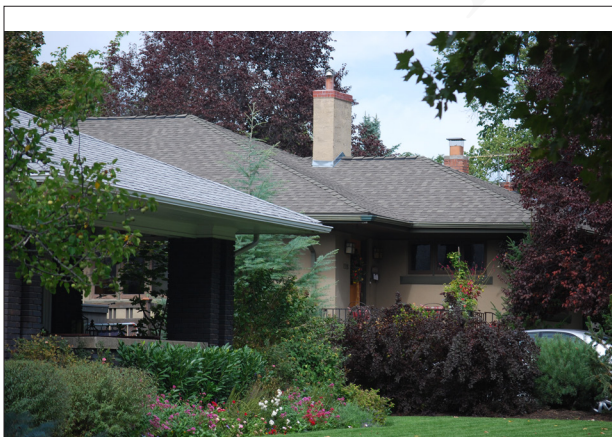
Horizontal lines and low roof profiles are a key characteristic of the bungalow styles and prompt designing an addition within and behind these profiles.
